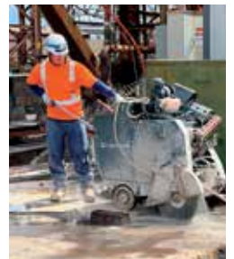
Concrete Cutting
